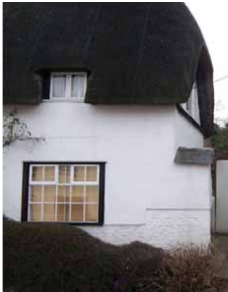
C - Church Street, Durrington Relevant design elements: - Timber casement windows - Render and whitewash - Thatched roof
