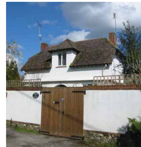
G - High Street, Durrington Relevant Design Elements: - chimneys - render - boundary wall
